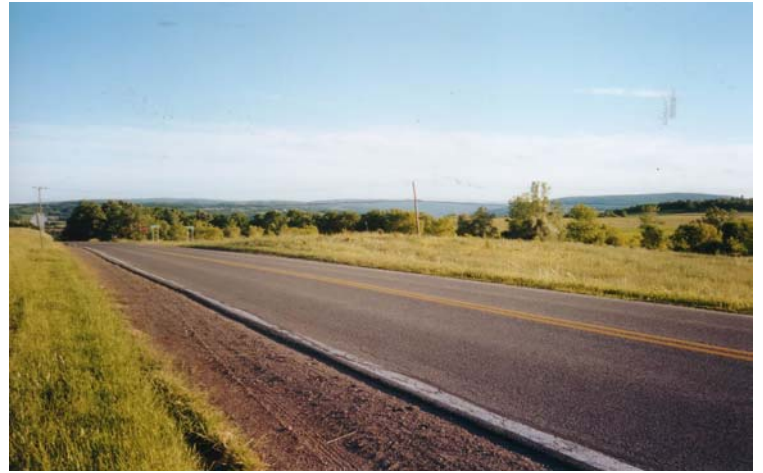
38. Baldwin Road near high school looking south
