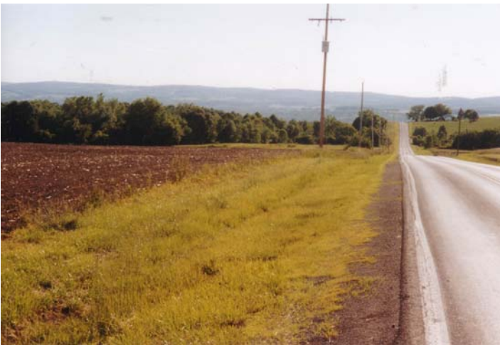
15. Lake to Lake at Middle Road looking west
